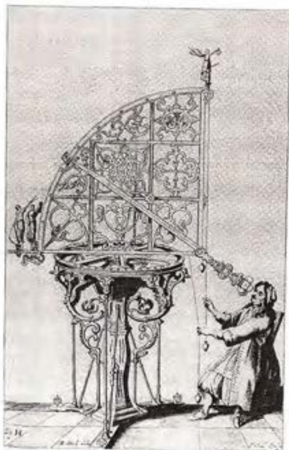
Johannes Hevelius observing with his azimuthal quadrant. From his Machinae coelestis pars prior (Danzig, 1673).
