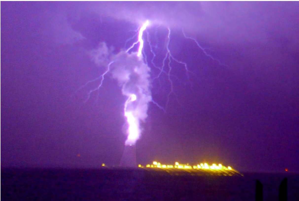
Figure 87: Lightning strike on the cooling tower of Salem nuclear plant (19 August 2011). (© Adapted from 'Eagle 9359'-Flickr). The contours of the cooling tower have been enhanced for better clarity.
