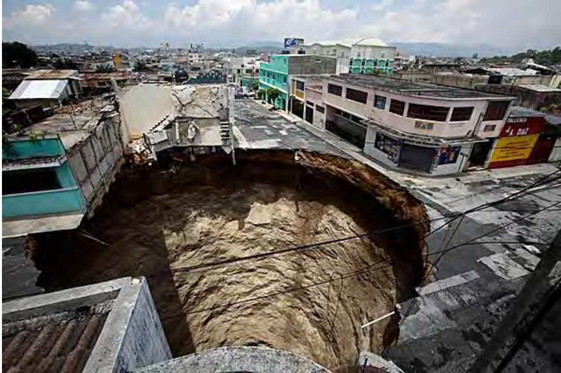
Figure 104: Picture of the giant sinkhole that opened up in Guatemala City, swallowing an intersection and a 3-story building on May 30 th , 2010. (© Reuters/Daniel LeClair)
