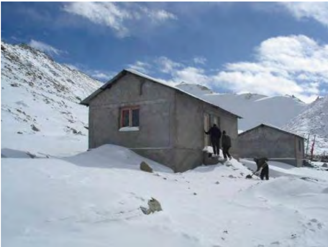
Figure 189: Above-ground buildings of the Chang-la seed vault. (© thehindu.com)
