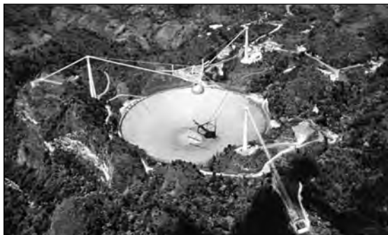
Figure 129. Built into a natural depression in karst limestone in Puerto Rico, the three-hundred-meter Arecibo dish is the world's largest telescope. It has often been used for SETI, and it appeared in the movie Contact . The sensitivity was calibrated on the Pioneer spacecraft, which still emits a feeble one-watt radio signal far beyond the edge of the Solar System at a distance of six billion miles. Arecibo could have detected a signal as weak as airport radar on planets around any of the eight hundred stars that Project Phoenix used it to search. In transmit mode, it can send a signal strong enough to be detected by an equivalent facility halfway to the center of the galaxy.
